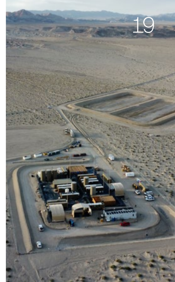
The demonstration project in Clayton Valley aims to showcase the proof of concept for sustainable technology production, using only 15% of the water, reducing emissions by between 60% and 80%, and utilizing 7% of the land compared to current practices.
